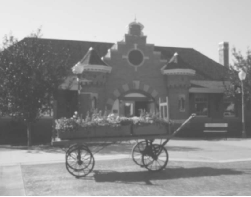
Evanston, Wyoming's, downtown revitalization efforts revolve around Depot Square.
